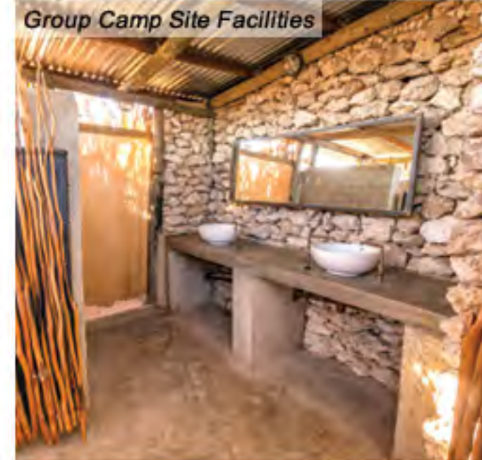
Group Camp Site Facilities
